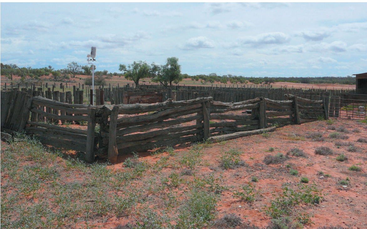
Figure 8. Belah Paling fence and Double Post-and-Rail fence on Nanya Station
